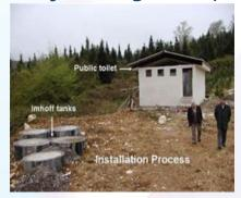
The project is designed to reduce waste water pollution entering Sefidrud River from a port town of 16,000, by using "Imhoff tank" technology. The reduction of 60% of pollution load is contributed to the preservation of surrounding national wetlands by the expected end of the project in June 2004.
