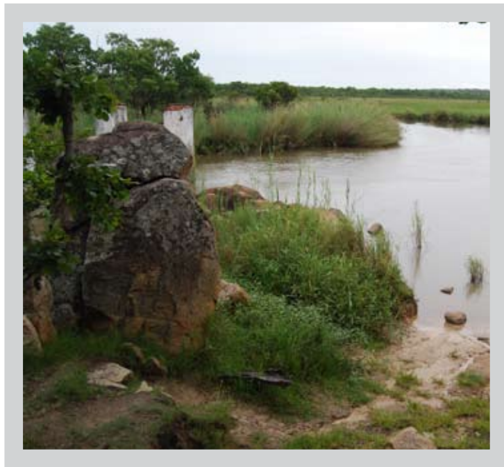
Damaged hydrological station, Rio Cuito, Cuito Cuanavale, Angola
