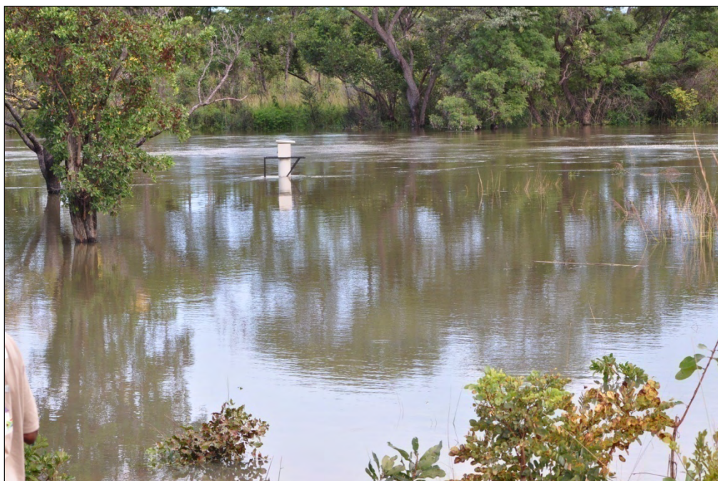
Figure 4-1 : Capico hydrometric station, on the Cueba River, flooded in mid-March 2009
