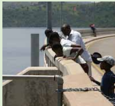
Steady, the Maguga dam wall is 115 metres high: reservoirs and careful coordination help avoid conflict over the Komati River's water.
