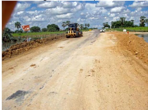
**Figure 3-11 : Construction in the north that partly contributed to flood damages**
