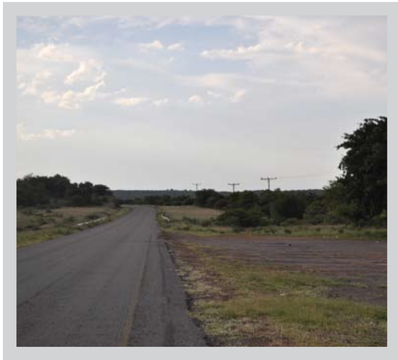
Paved road in Botswana part of the Basin, 2008
