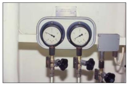
Figure 4. Pressure meter of ships ballast water pump.
