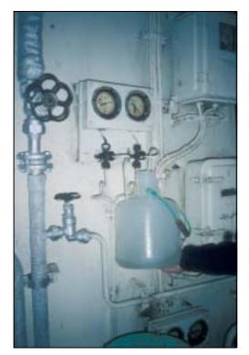
Figure 1f. Collection of samples from bleed valve in a ship's engine room.
