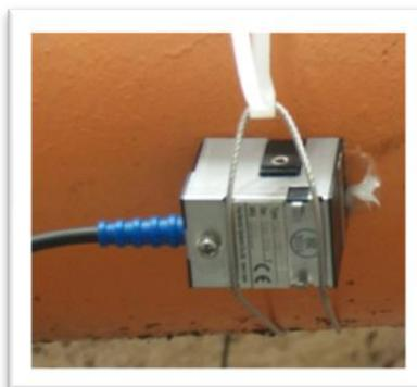
**Figure 9. Flow Meter Transducer**
