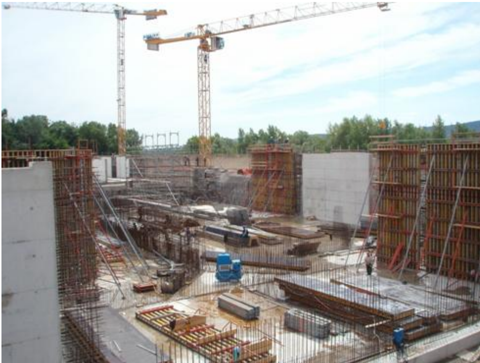
Construction of the new aeration tanks: concreting
