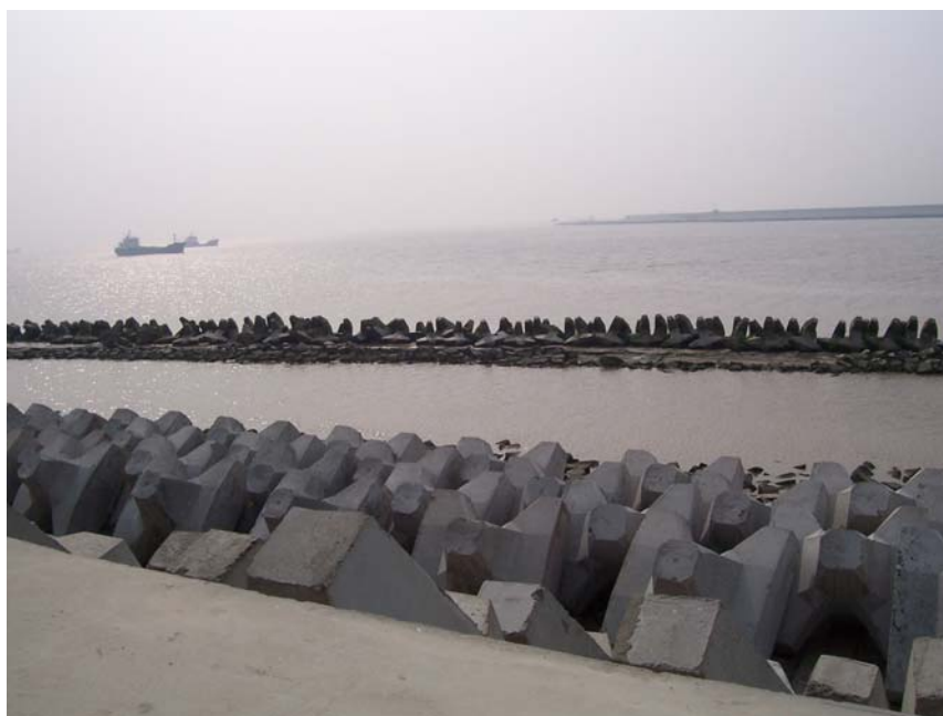
Photo 2 – Dykes along the Yangtze coast, to prevent from coastal erosion being raised from reducing sediment budget, typhoon and high tides.
