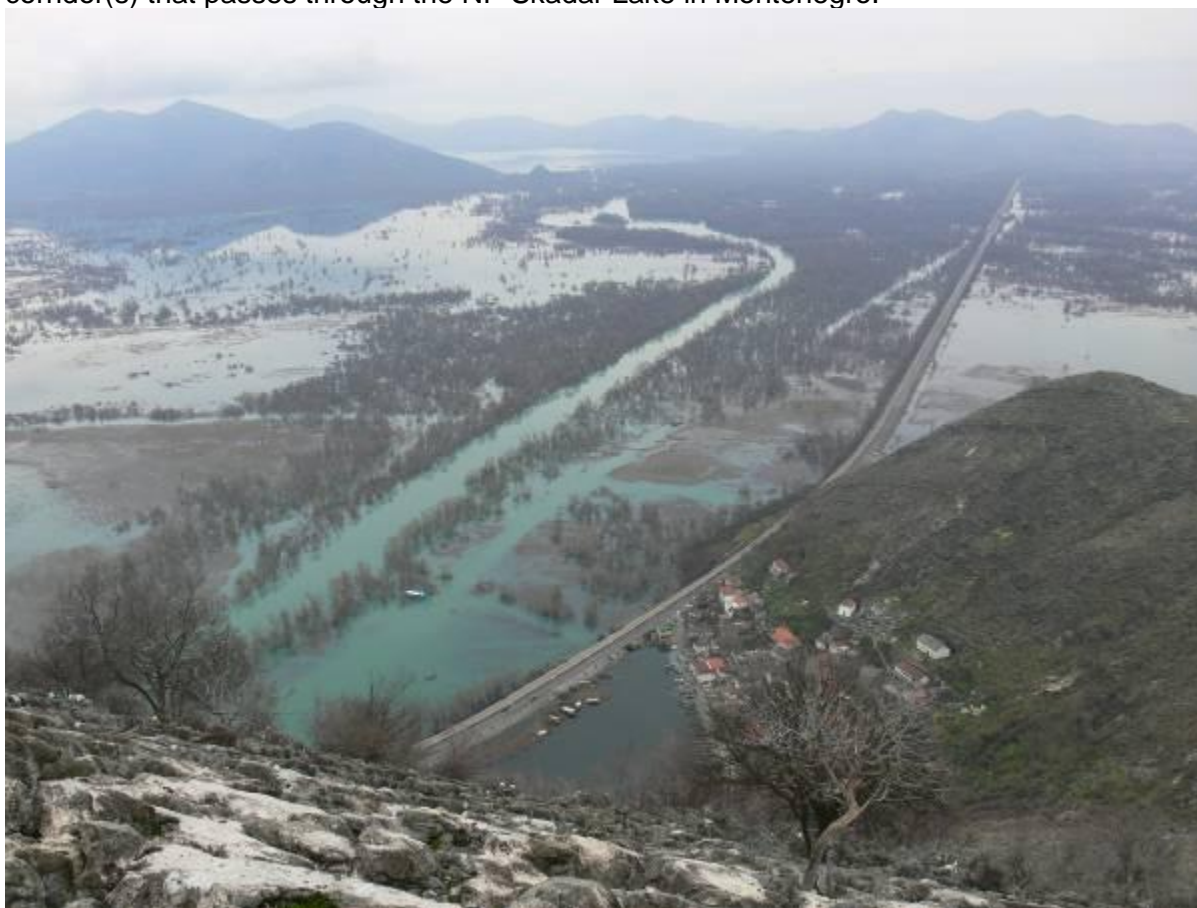
Embankment for existing road and railway is crossing NP Skadar Lake
