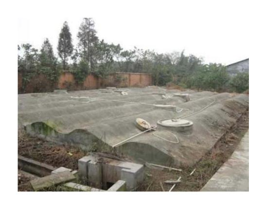
New-typed big biogas engineering (with parallel separated fermentation reactors and gas storages) can reduce construction costs by a big margin.
