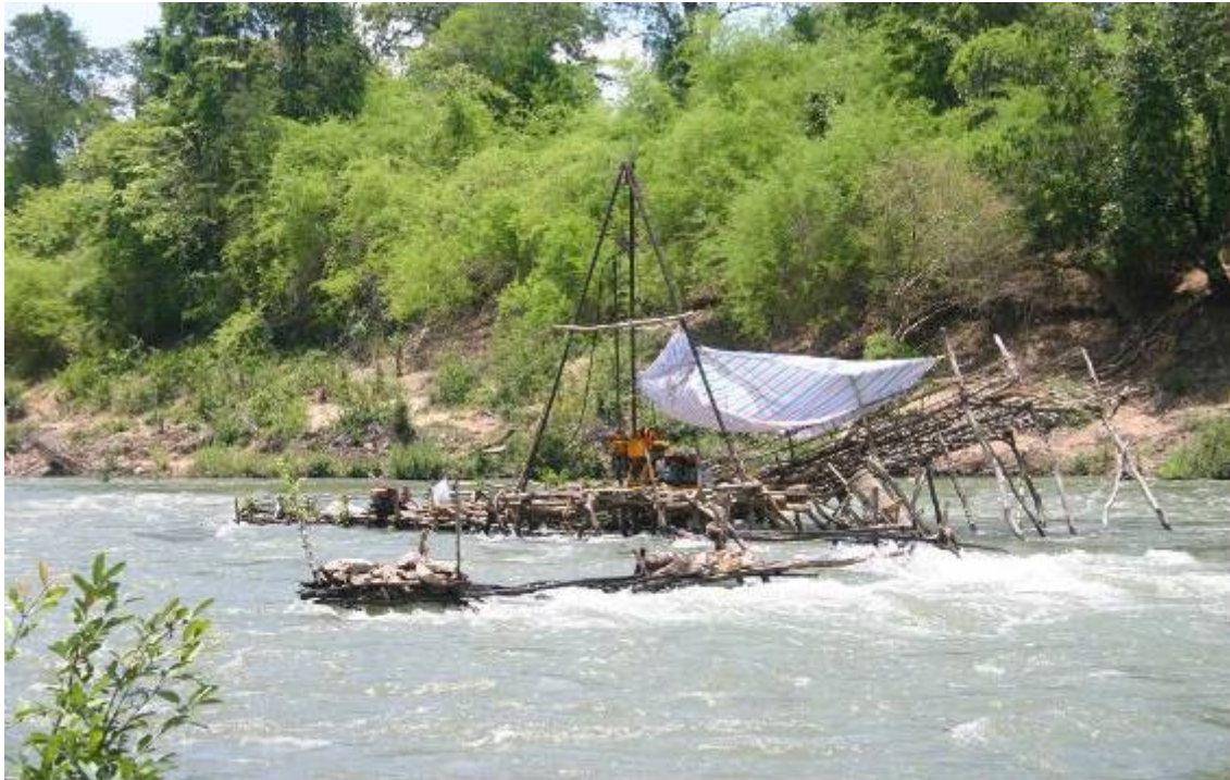
Hou Sahong – drilling rig for dam survey
