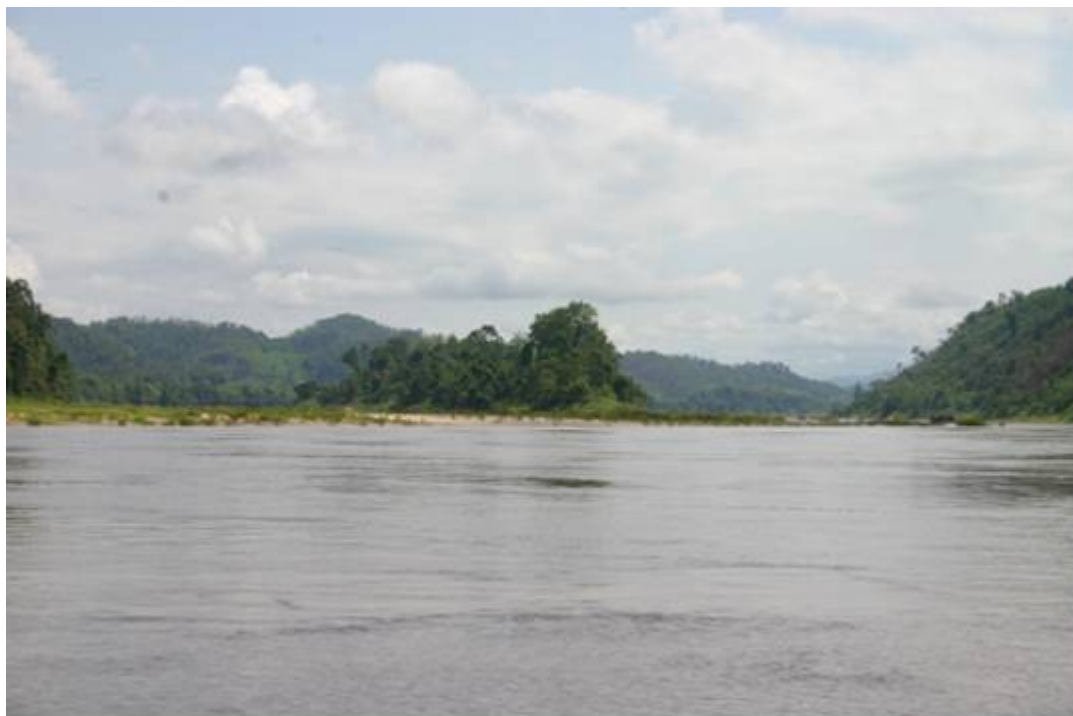
Pak Lay Dam Site Option 1 – looking upstream
