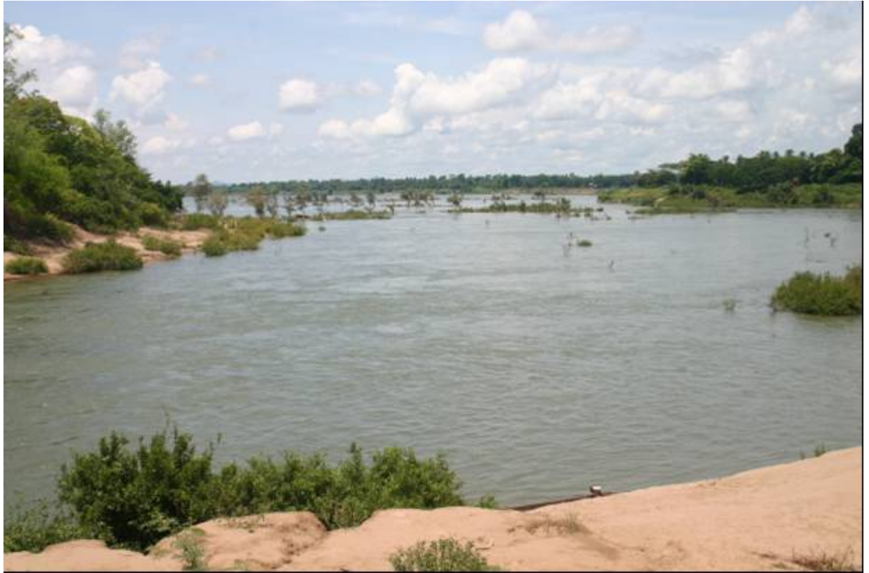
Dam site looking downstream
