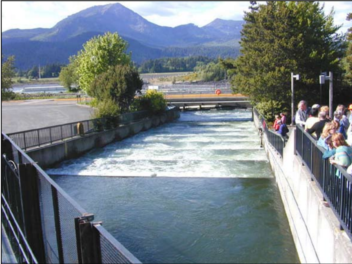
Fish ladders, such as the one pictured above at Bonneville Dam on the Columbia River, are one of the many mitigation mechanisms used in an attempt to reduce the barrier effect on fish migration in America's largest river. These, however, are generally not applicable to hydropower dams in the Mekong.
