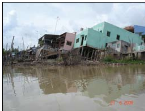
Plate 7. Severe to total structural damage caused by riverbank erosion and soil saturation during flood conditions (Dong Thap province).
