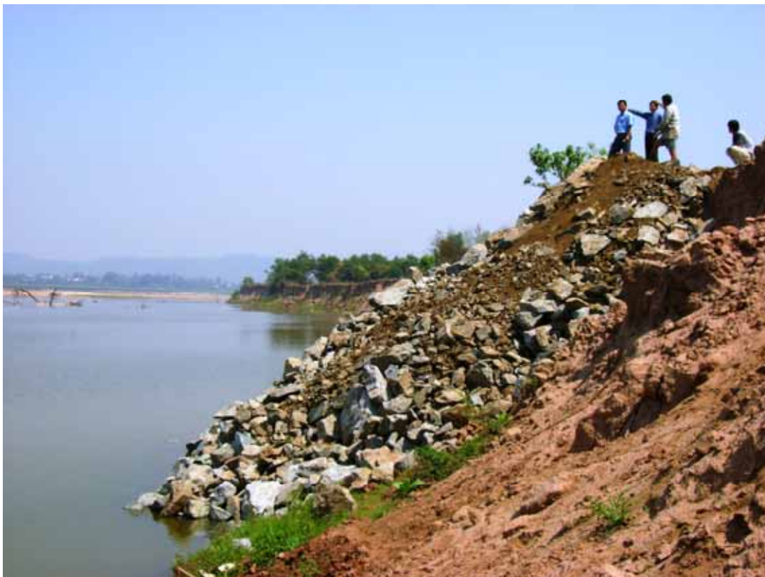
Figure 3.9 Hardpoint constructed along the Mekong for controlling riverbank erosion.
