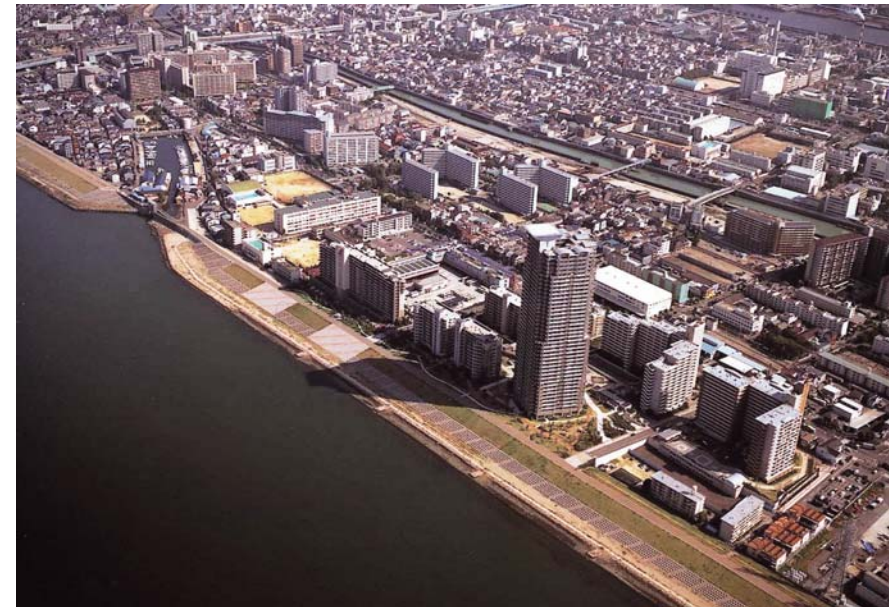
After levee construction
