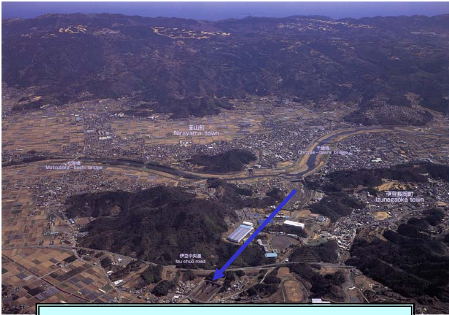
Kano River Floodway (Shizuoka Pref.)
