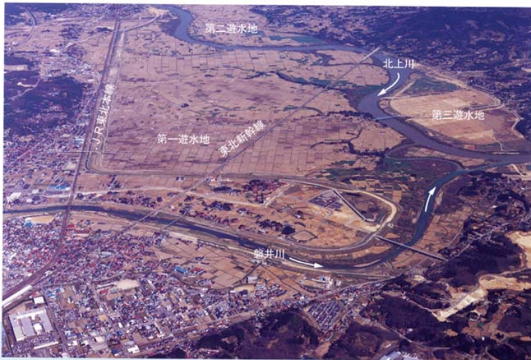
Ichinoseki Detention Basins
