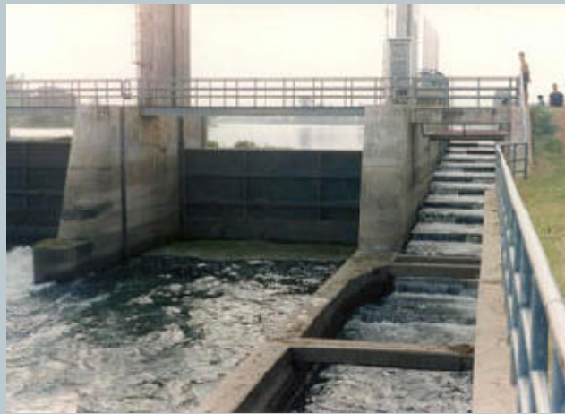
Fishways allow some fish species to swim past constructed barriers
