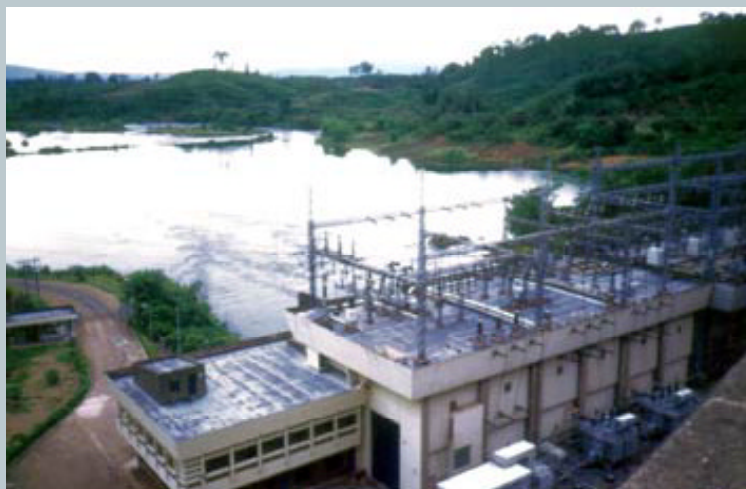
Nam Ngum hydropower dam, in the Lao PDR
