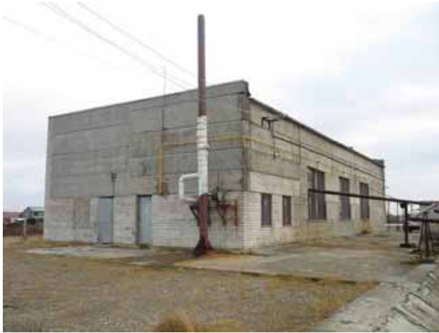
Photo 1. Building of the Bondarny WWTF, view from the water discharge point
