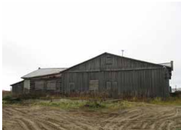
Photo 2. Kachgort WWTF, view from the sludge pit
