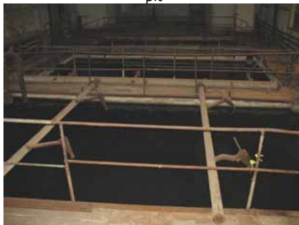
Photo 4. Kachgort settling tanks
