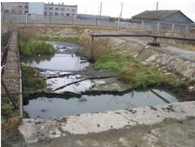
Photo 3. Sludge beds of the Bondarny WWTF
