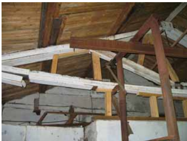
Photo 5. Kachgort WWTF, ceiling beams
