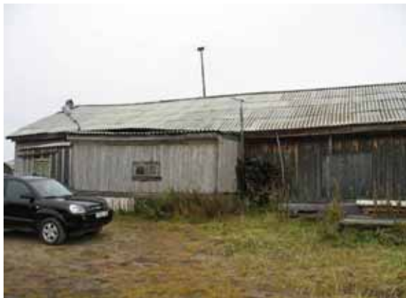
Photo 1. Kachgort WWTF, view of the entrance
