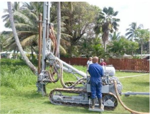
Drilling groundwater monitoring wells in the demonstration project area
