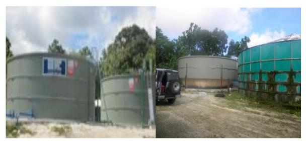
**Figure 9:** The two new 240 kL storage facilities at Alofi South
