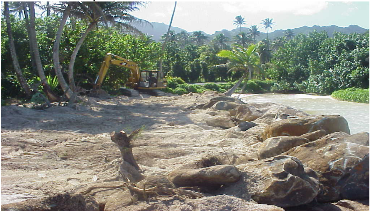
Photograph 5.0: Land preparation on the foreshore area
