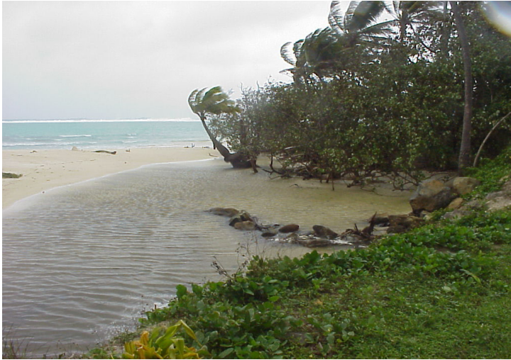
Photograph 13.0: Another example of an attempt to construct a coastal protection structure.
