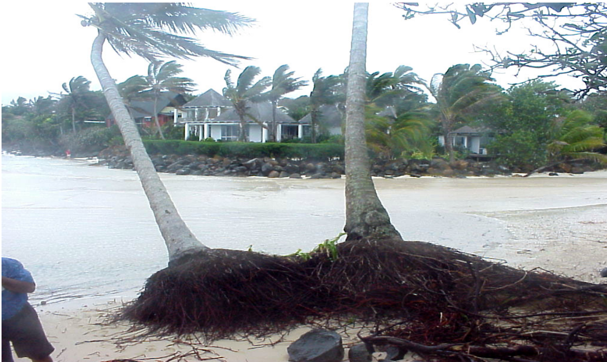
Photograph 3.0: Rock revetments in the background has resulted in the degradation of adjacent properties.
