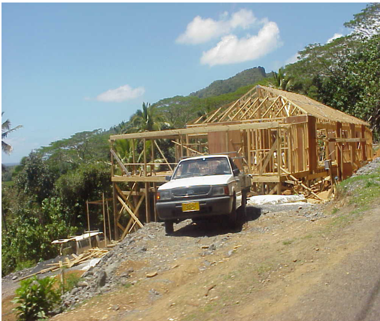
Photograph 5.0: A typical work site on sloping lands.
