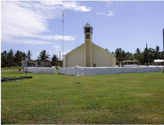
Liku Church Building
