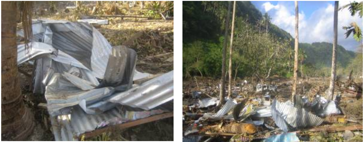
General conditions of Iron Roofing Materials at the affected areas
