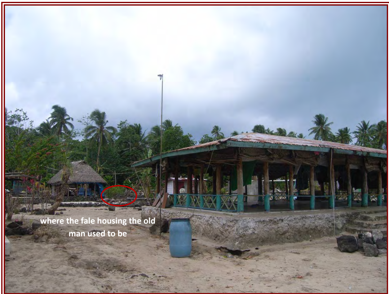
Figure 31: The set of fale at Lepuia'i where the front open fale prevented the old faleoo in the middle from being washed out to sea by the backwash of the waves
