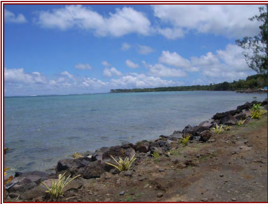
Figure 5: A seawall found at Satoa made up of various volcanic rocks and mortar lined the coast
