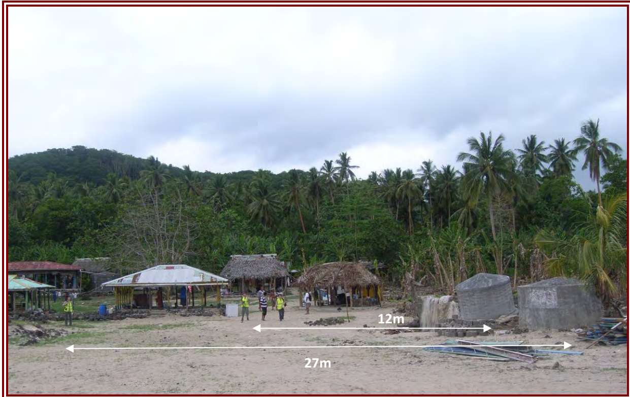
Figure 29: Two water tanks moved were lifted from their very thin concrete screed foundations 12m and 27m respectively
