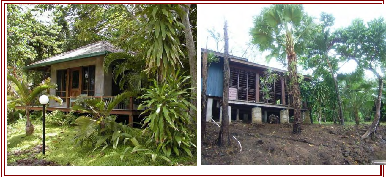
Figure 14: Photo taken from the www.preferencetravel.co.uk website of the Sinaeli Reef Resort of the dense forested area before the tsunami (left) and the same location with exposed foundations after (right)
