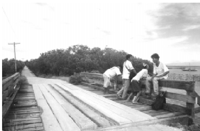
Figure 3.9. Protection plantation established to protect causeway of Pangangan, Calape, Bohol.
