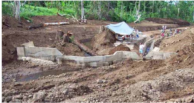
Figure 4-1 – Alaoa Hydro Intake Being Cleaned and Repaired Following Cyclone Heta, 2004
