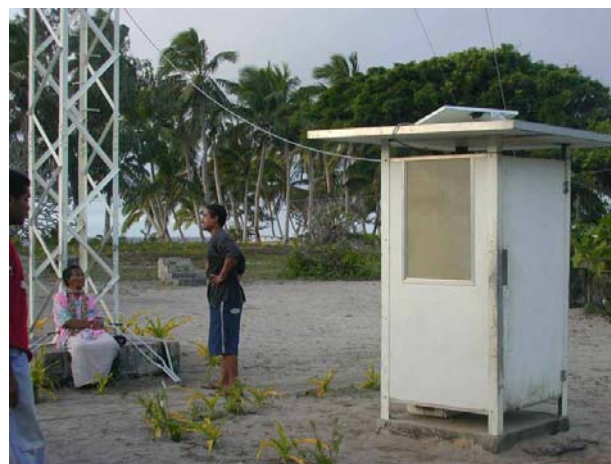
Fig 4.6 - Mango Island PV powered phone
