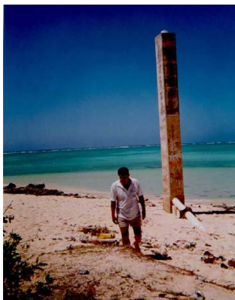
Tarawa, Betio Outfall showing Ventilation Pipe.
