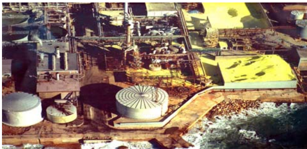
So 2 storage at Chemical Lebanon (North).
