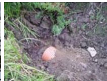
drainage system & sprigs fenced
