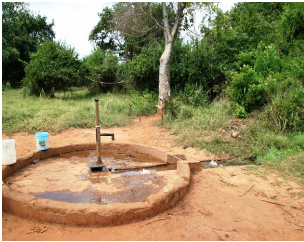
Figure 14: A well constructed in cooperation between TASAF and Kilwa local communities, Aug 2010
