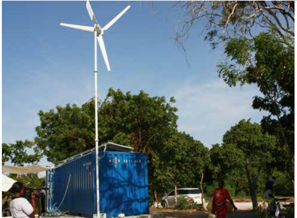
The UNIDO supported Water purification plant utilizes wind and solar energy (Photo: COAST Project)
