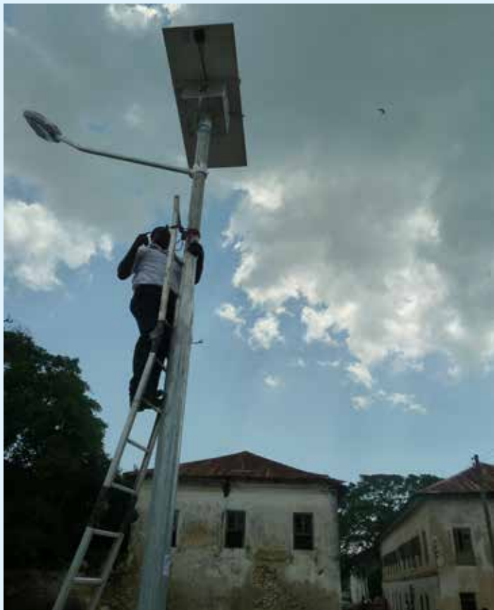
Installing the solar lights in Bagamoyo, an activity under the EMS/TEST thematic area (Photo: COAST Project)
