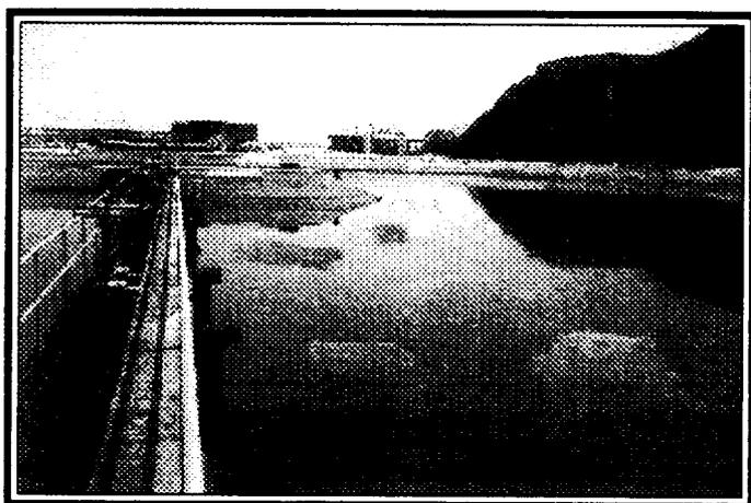
Fig. 4. Last step in oilwater separation lagoon. Note patches of oil on the water.
