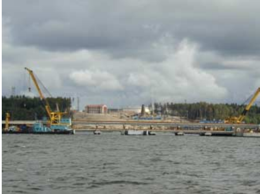
Figure 2. Primorsk oil terminal under construction in autumn 2001.
