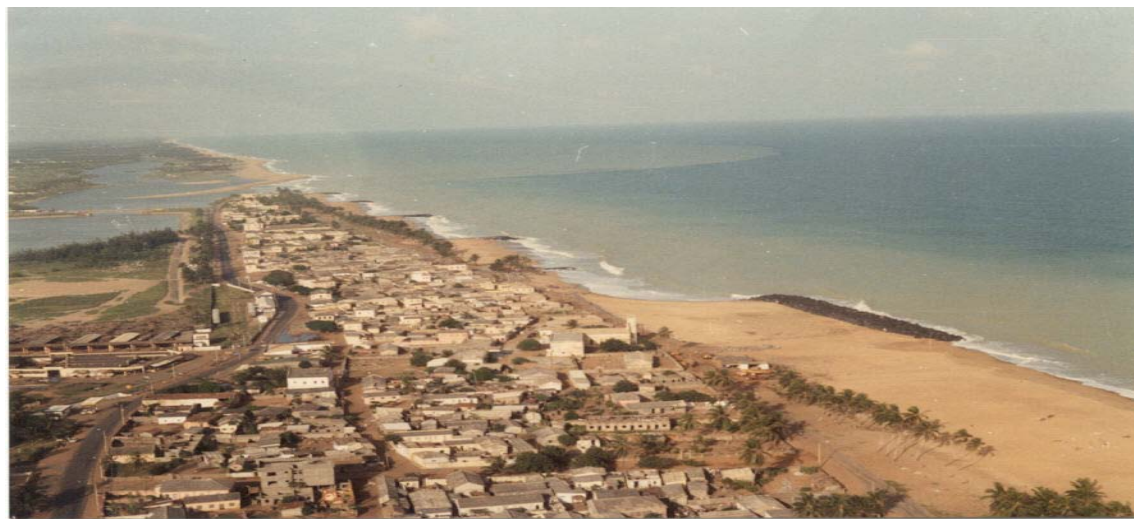
Figure 5. Coastal protection measures in Togo.
