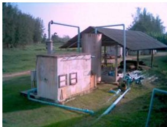
Biogas Purification Unit
