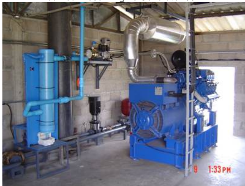
Biogas Generator 230 kw
