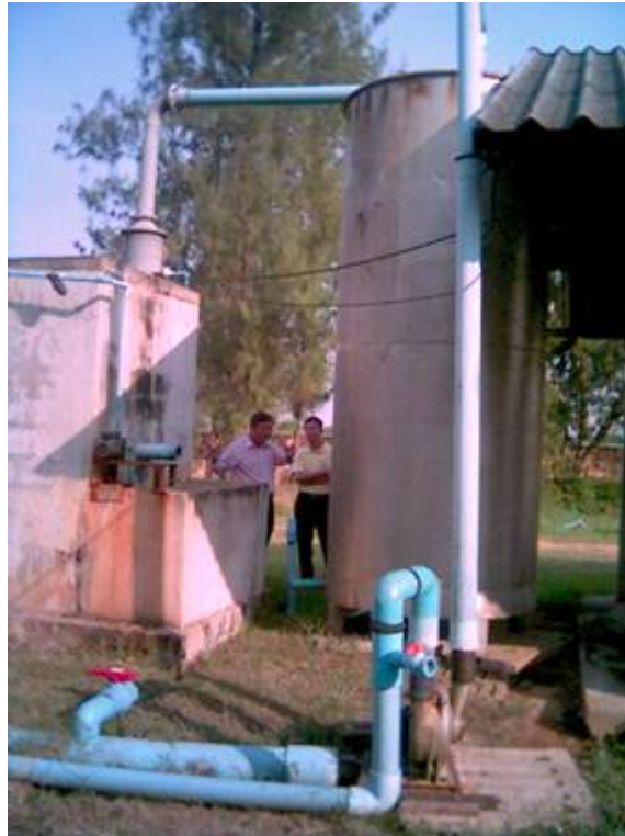
Biogas Purification Unit ( Biological Treatment)
