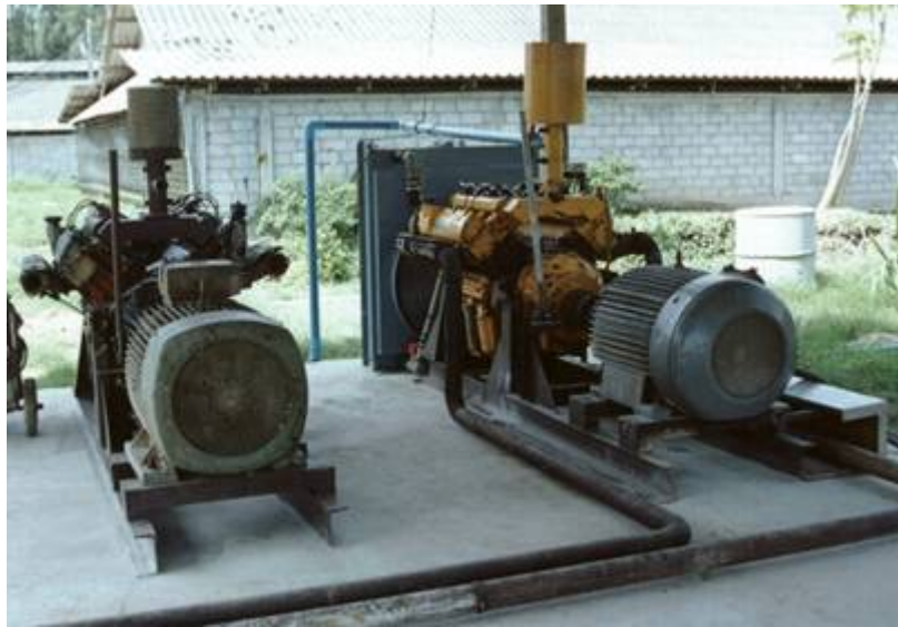
Modified Diesel Engine Generator 90 kW
