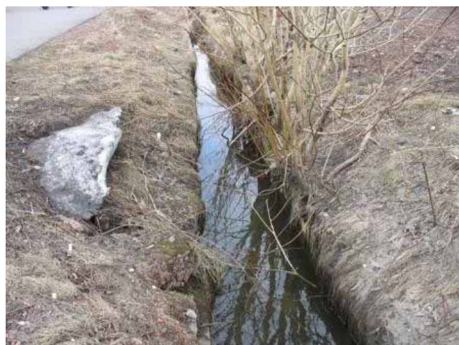
Photo 10. Chutes for surface water withdrawal
