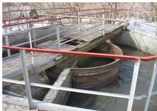
Photo. 5. Sand traps with rotary movement of water
