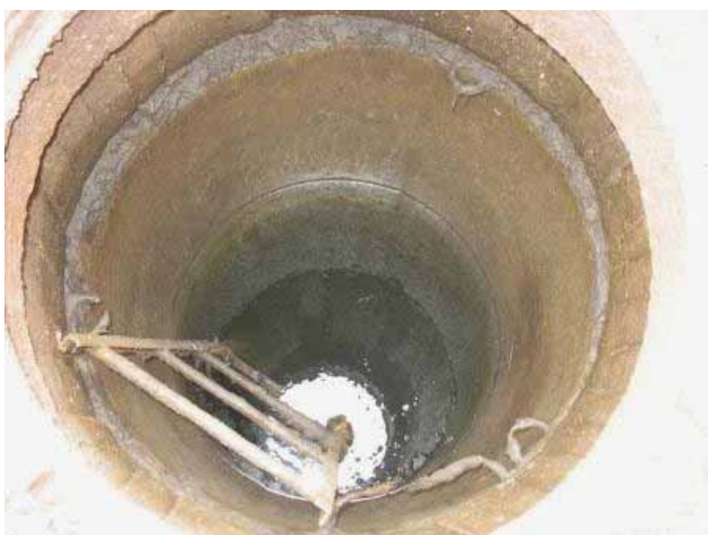
Photo 3. Network well with backwater
