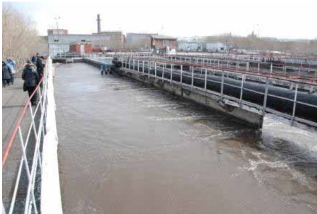
Photo. 3. Passage active sludge tanks
