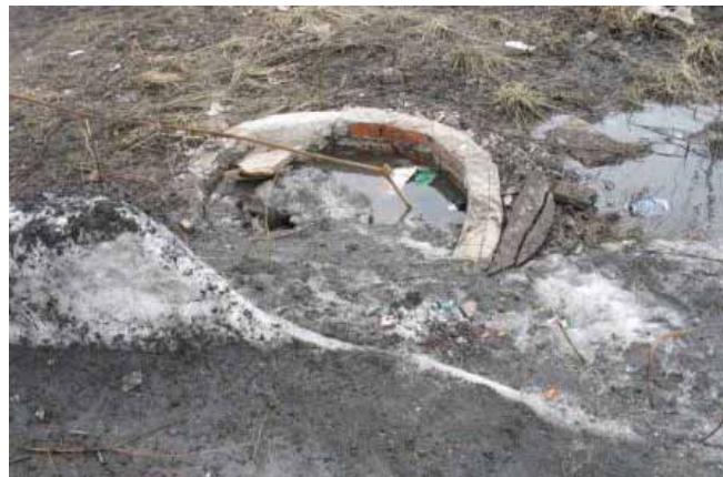
Photo 2. Well filled with water and without floor slab
