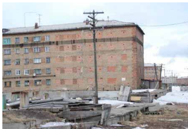
Photo. 8. Partially blocked dwelling house
