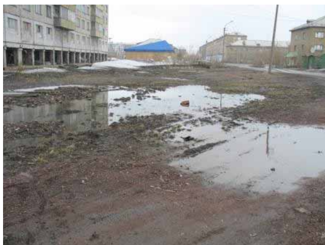
Photo 9. Area of the Zheleznodorozhniy district where sewage system is located
