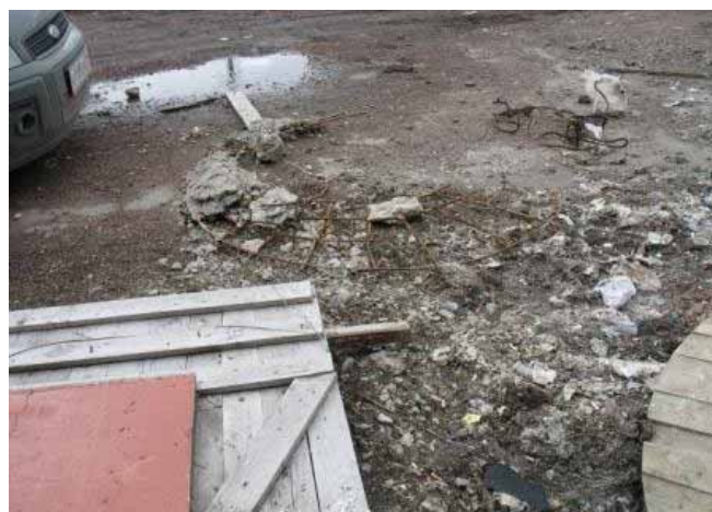
Photo 8. Demolished floor slab
