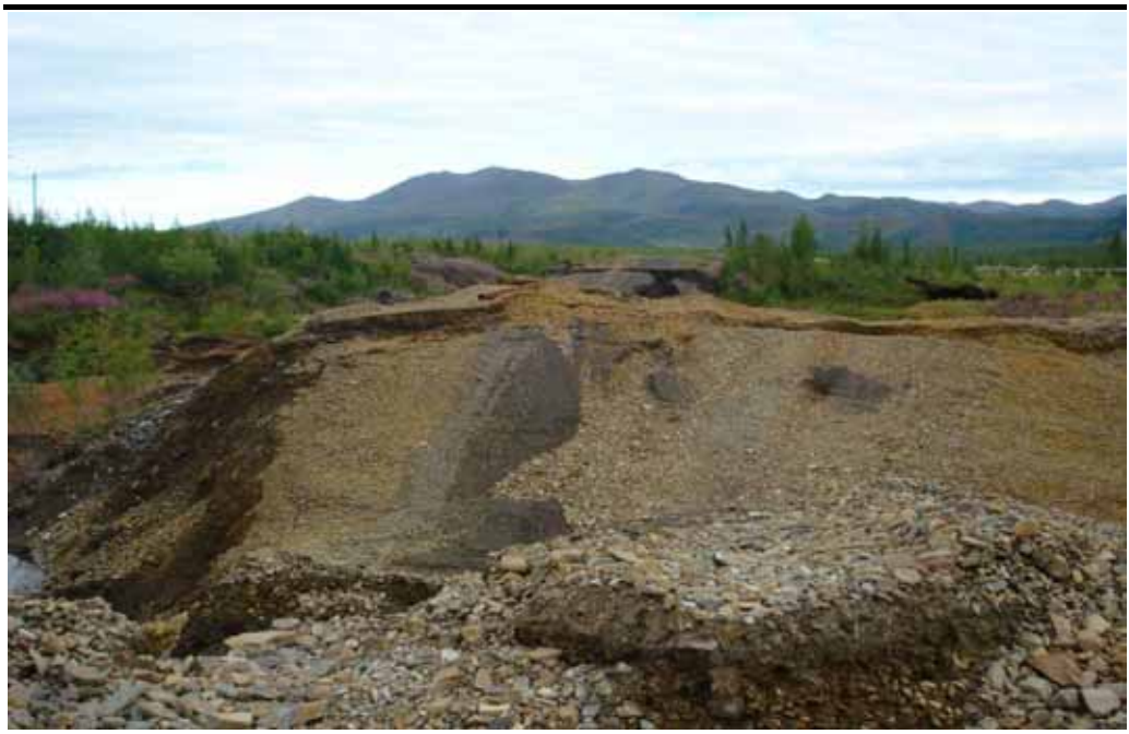
Photo 13 Access road section subsided as a result of a washout. Photo 2
