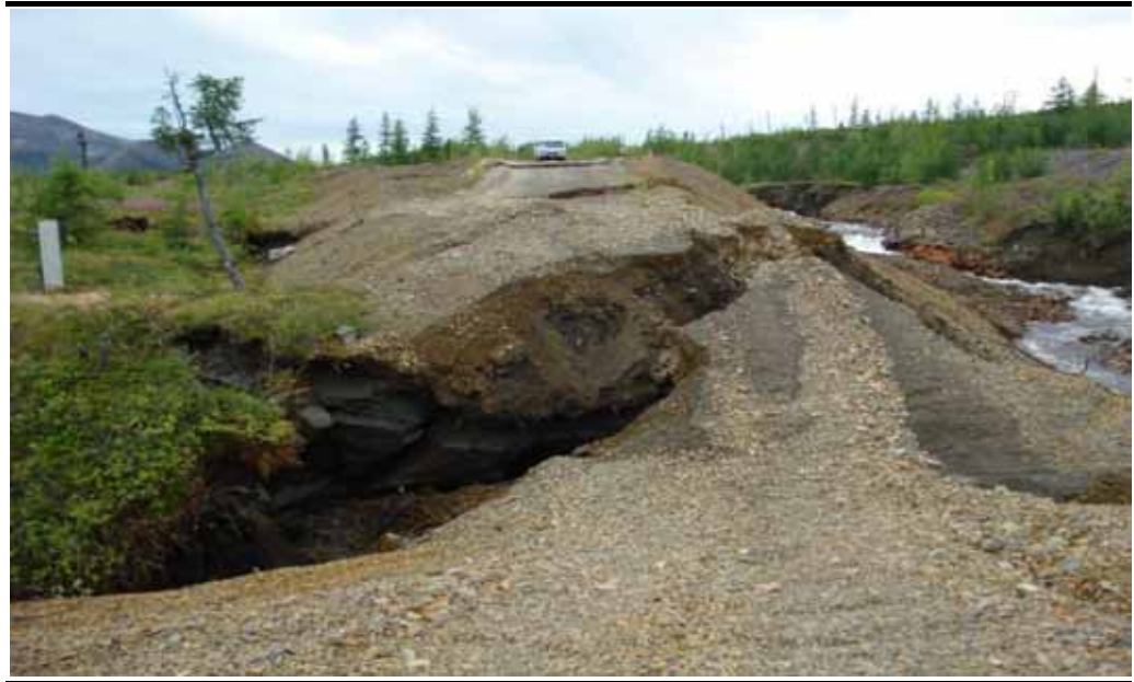
Photo 15 The point where the Poiskovy Stream disappeared under the road. This part of the road was just covered with crushed stone; the embankments and the dam had not been reinforced with concrete slabs.
