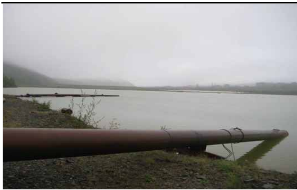
Photo 4 Due to the corrosive medium of the tailings pond, the siphon tube (8mm thick) abstracting water from a depth of 1.2m deteriorates completely within 1.5 to 2 years.
