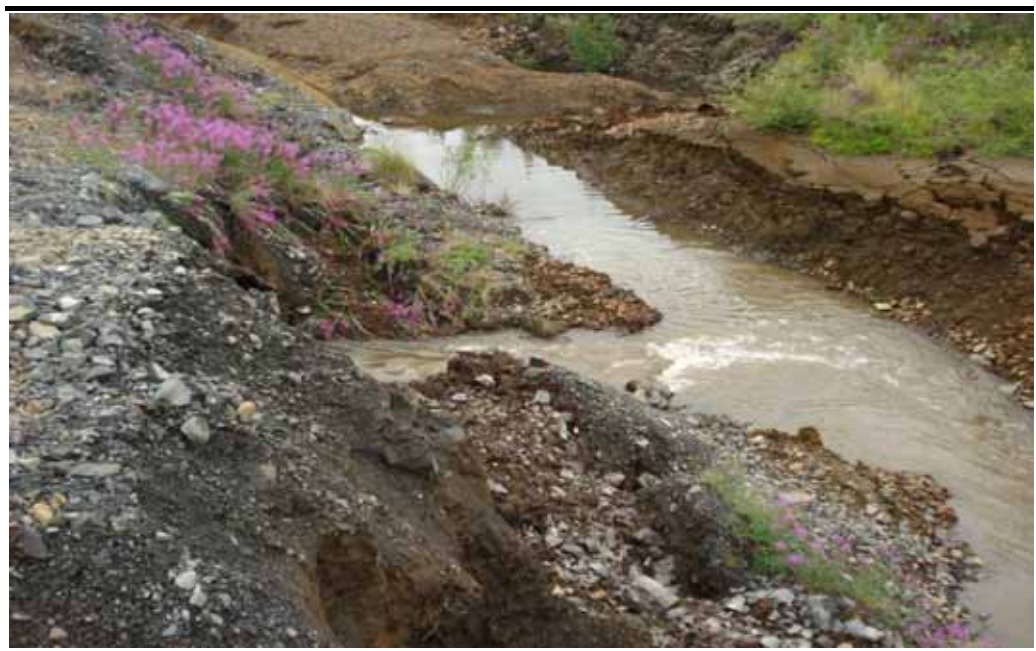
Photo 15 The point where the Poiskovy Stream disappeared under the road. This part of the road was just covered with crushed stone; the embankments and the dam had not been reinforced with concrete slabs.
