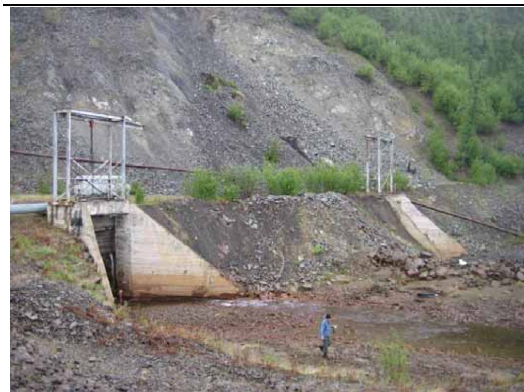
Photo 7 The area of discharge of wastewater from the ash disposal area of the boiler station adjacent to the tailings. There are no wastewater treatment facilities at the boiler station.
