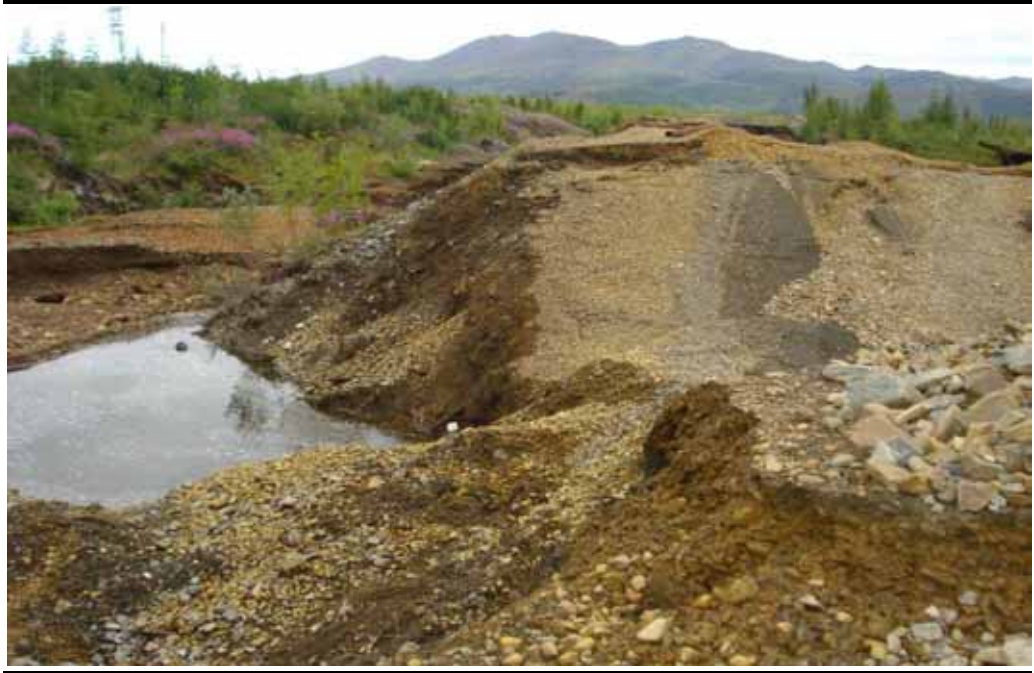
Photo 13 Access road section subsided as a result of a washout. Photo 2
