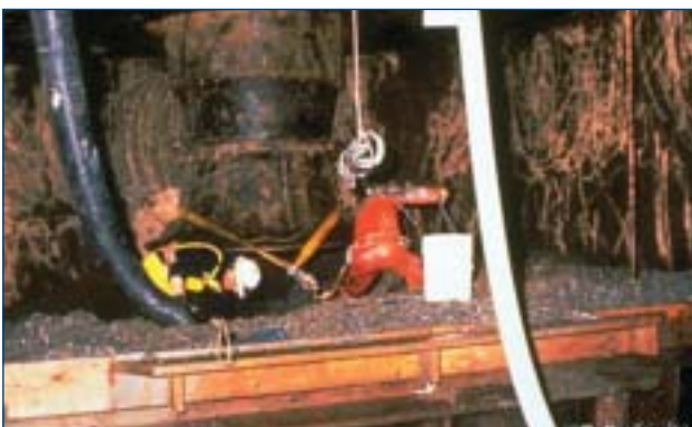
Workers clearing Zebra Mussels from power station water intakes – Detroit (Source: R Peplowski).
