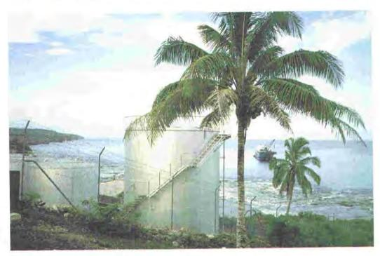
The bulk fuel store at Alofi is not only vulnerable to cyclones but its position means that any accidents lead to a high likelihood of petroleum being spilt into the sea.
