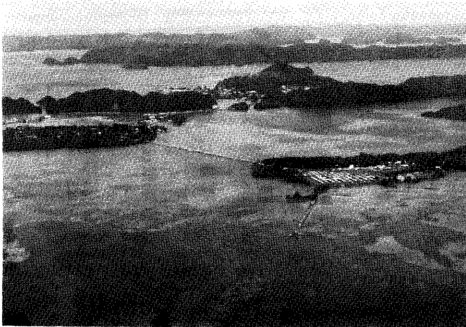
Plate 4: A network of causeways connecting Koror to nearby islands. In the foreground (bottom right) is Arakebesan Island with Belau National Hospital, the Presidential residence and Palau Telecom. Ngermalk and Malakal wharf are top centre.
