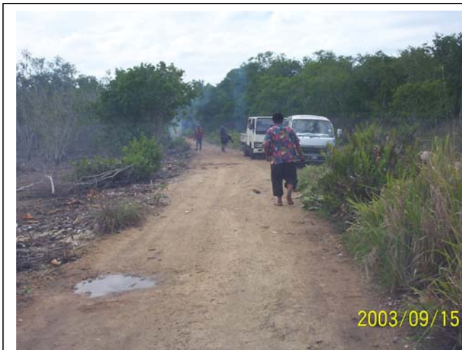
A great job almost done!
