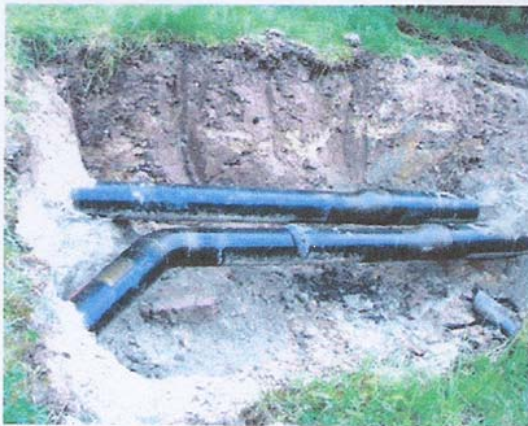
Preparation of Pipelines for wall thickness gauging
