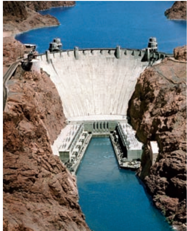
FIGURE 5 THE HOOVER DAM ON THE COLORADO RIVER, USA.
