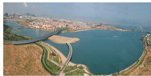
The view of Wuyuan Bay in 2008 after restoration
