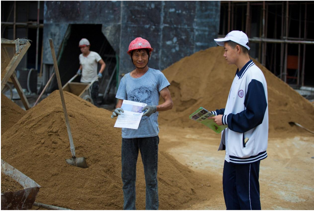
The students presented a leaflet to the construction worker about bird protection
