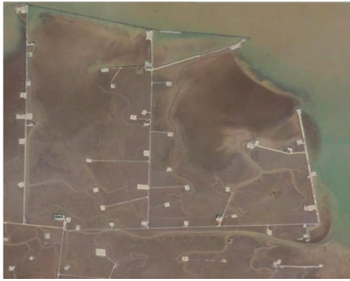
(a) Oil exploration infrastructures in Yellow River delta
