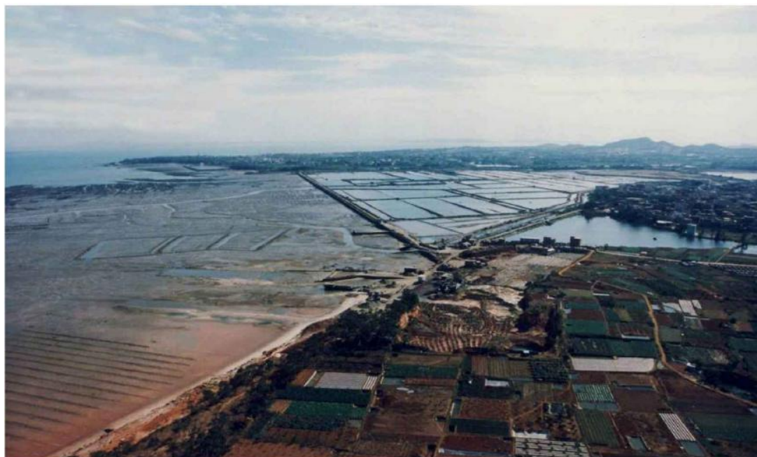
Fig. 1.2 Poor hydrodynamic condition in Wuyuan Bay
